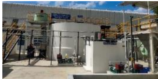
Sludge storage tank
