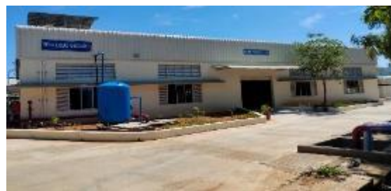
Chemical storage Room
